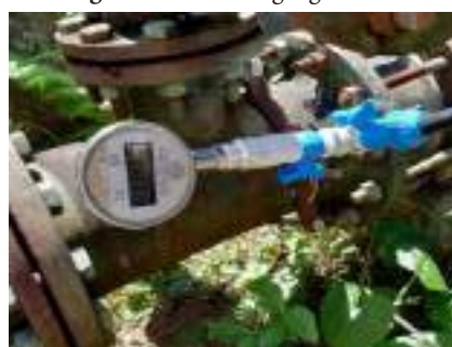
Figure 4 - Pressure gauge socket
